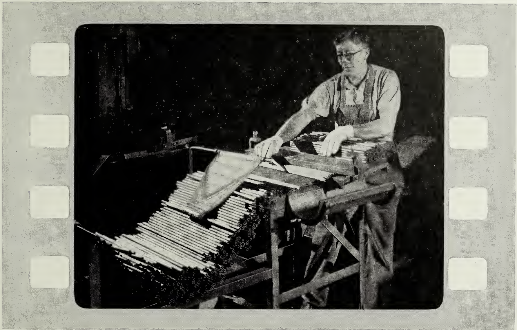
"National" projector carbons receiving straightness test
